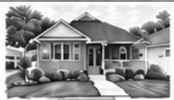
222 Coolidge Place — Built 2000
