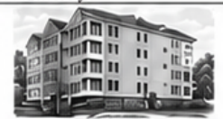
Radcliffe Court — New Construction
